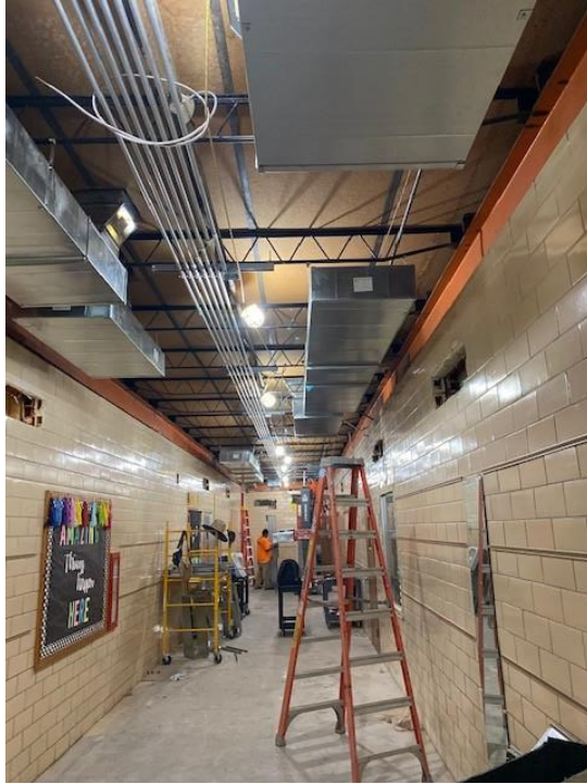
Corridor HVAC and Electrical Rough In
