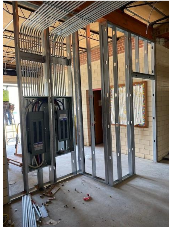
Electrical Rough, Secure Entry
