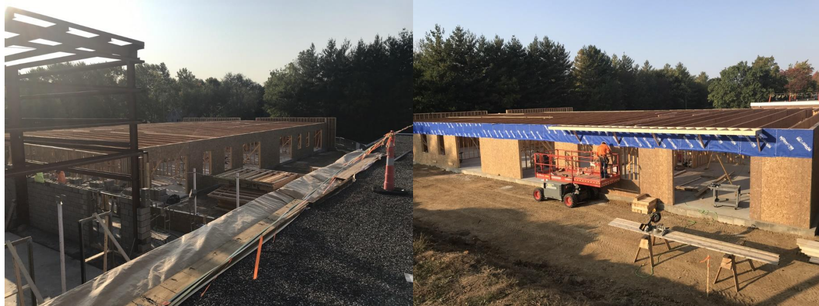
Classroom Addition Shell Ongoing
