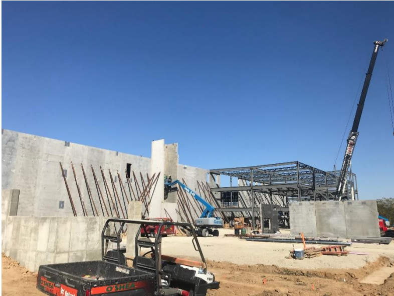
Starting Kindergarten and Kitchen Structure
